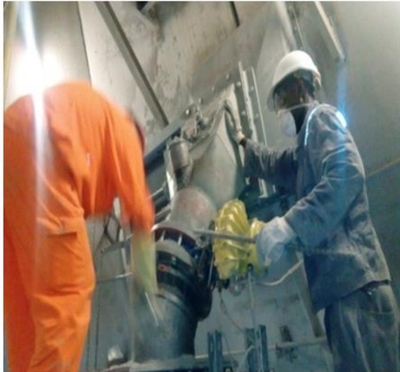
Figure 9: Cement silo (caked cement) cleaning
