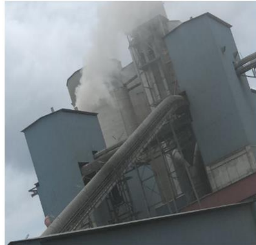
Figure 10: High cement dust emissions
