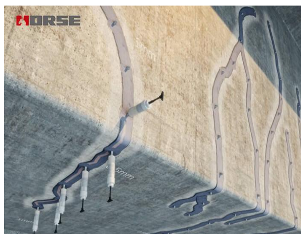
Figure 14: Repair of a building beam using epoxy injection [30]
