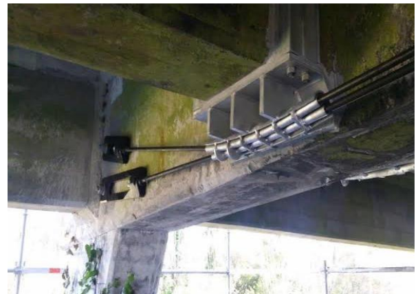
Figure 13: Post tensioning on the beam of a structure [28]
