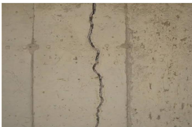
Figure 2: Vertical structural crack on column [12]
