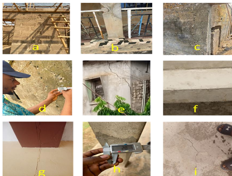
Figure 16: Some of the cracks observed and recorded
