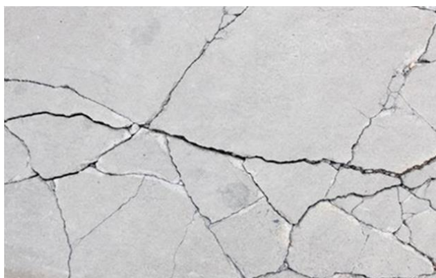
Figure 1: Non-structural shrinkage crack [9]
