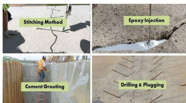
Figure 15: Some repair methods for structural cracks on building [38]
