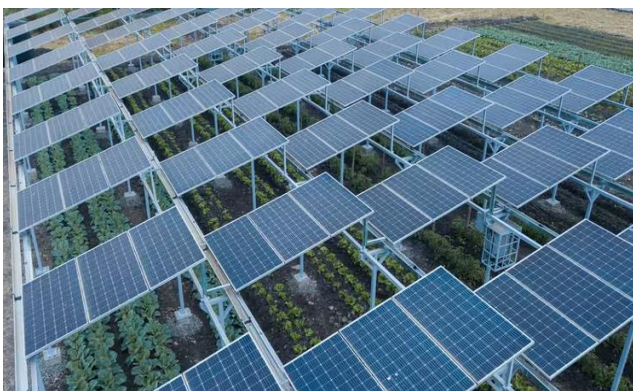
Figure 7: Illustration of agrivoltaics pilot system showcasing the integration of solar power generation, crop cultivation, and rainwater harvesting within a unified land area [49]
