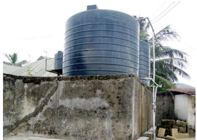
Figure 1: An elevated concrete water stanchion.
