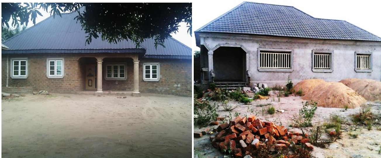
Figure 1: Three bedroom bungalows constructed with Makurdi local burnt bricks (a) without rendering; (b) with rendering
